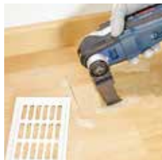
Plunge cutting in laminate, e.g. for installing a ventilation grille
