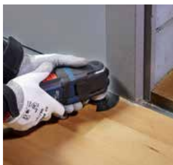
Cutting out laminate/parquet accurately, e.g. for installing a ventilation grille
