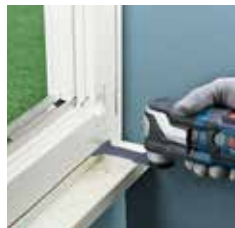
Plunge cutting in wood or metal, e.g. for removing window frames or door frames
